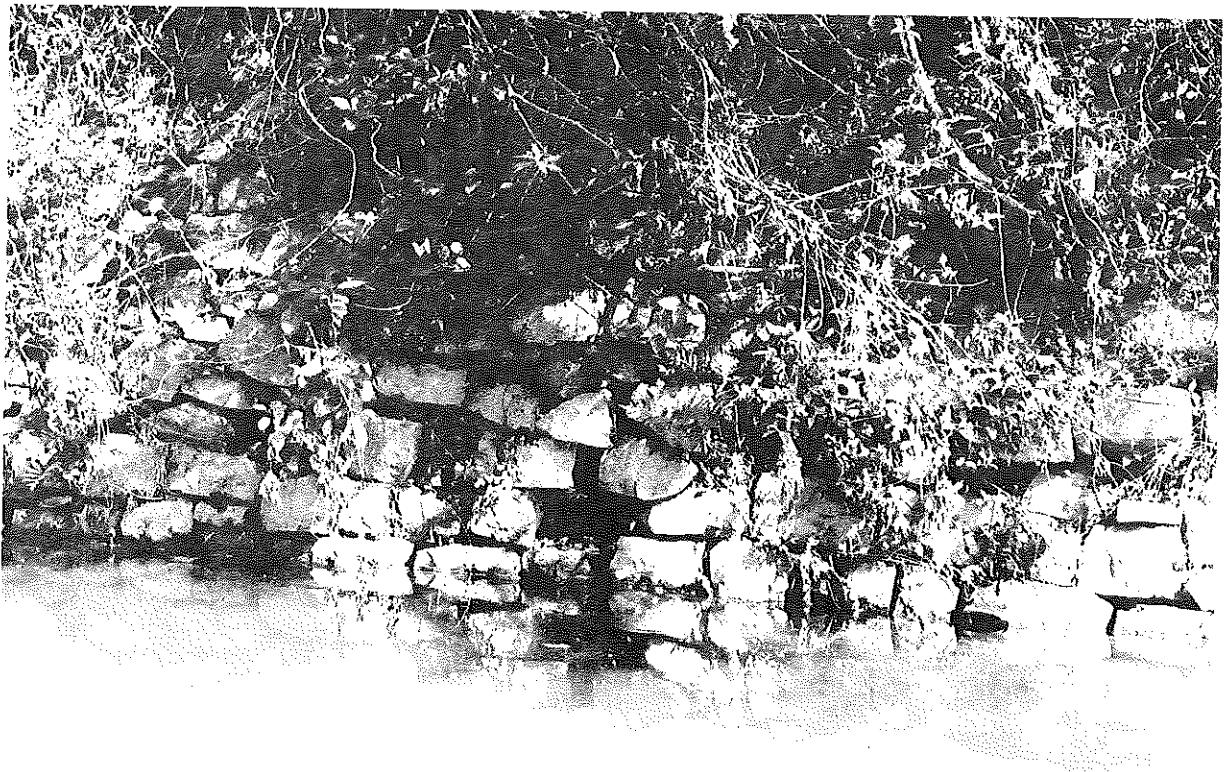
The stone lining of the canal's bank, called rip-rap, is a constant reminder that the canal is a 19th century man-made artifact. Above, near Stockton.
